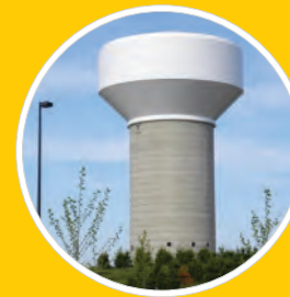
Overhead Water Tank
